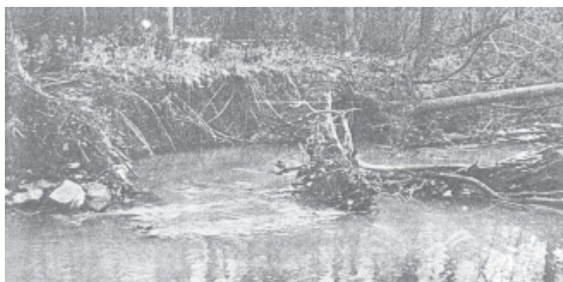
Fig. 17.6: Stream bank erosion
